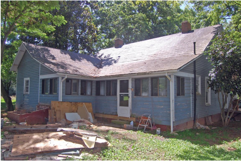
Latta Family House, Rear (North) Elevation and Kitchen Wing, Looking South.
