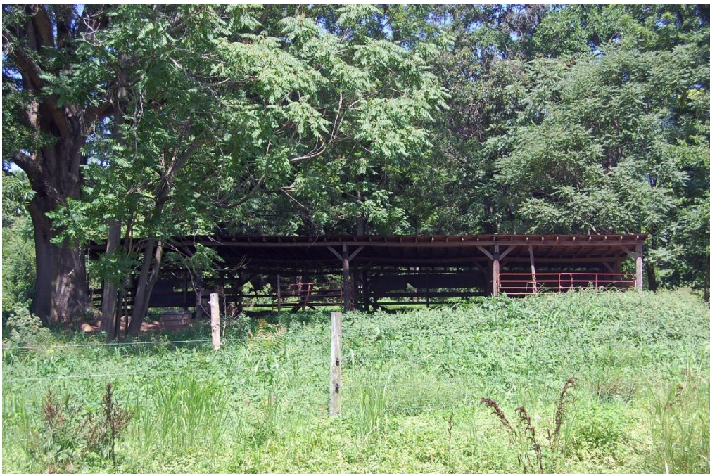
Latta Family House, Livestock/Equipment Storage Shelter, Looking West.
