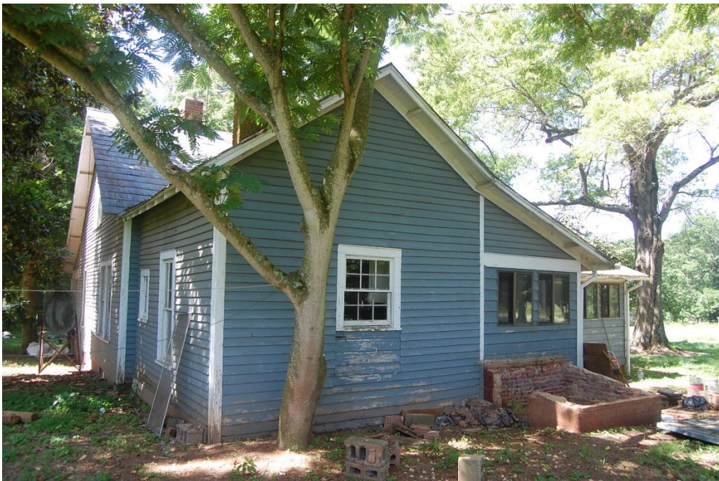
Latta Family House, Rear (North) Elevation of Kitchen Wing, Looking South.
